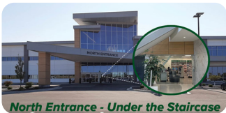
North Entrance - Under the Staircase
